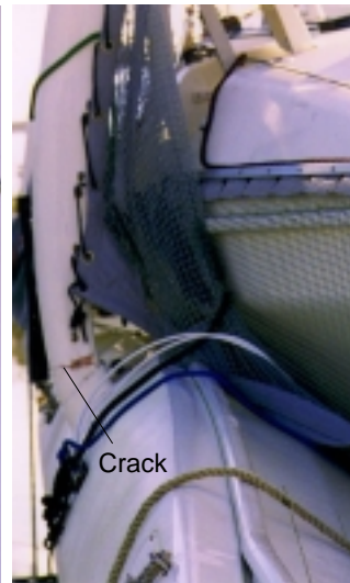
...then fwd. beam may also be damaged (see crack on fwd. side)
