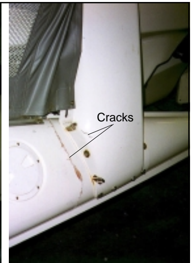
Aft beam damage - note also large crack running around float deck
